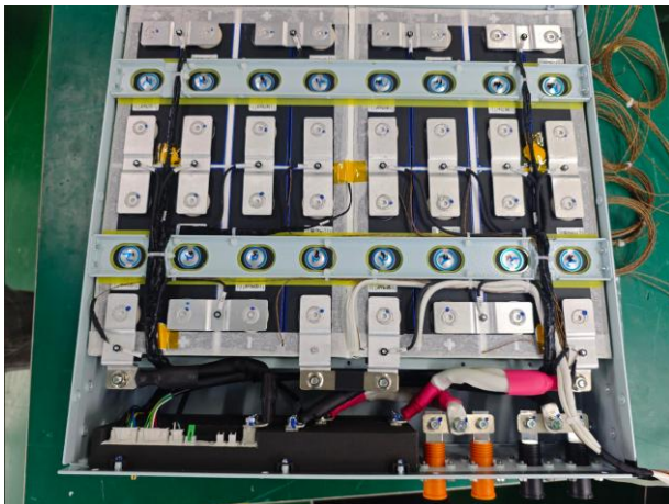
Figure 8 - Photo of module – Internal view
